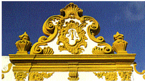
A typical painted façade
